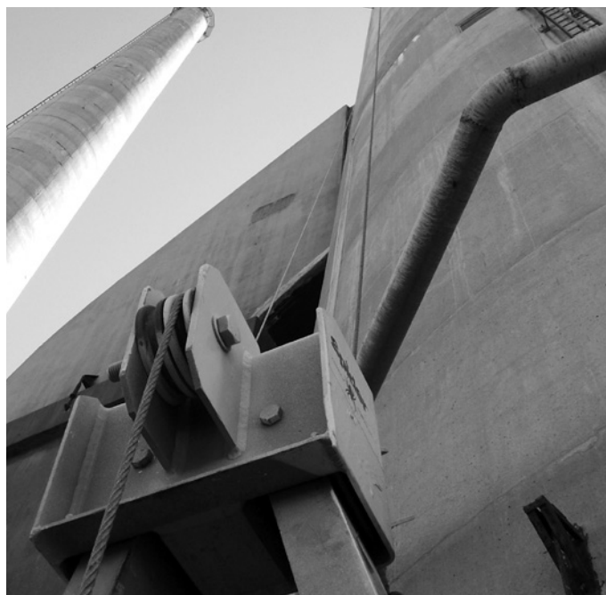
Pin-style sheave connection reduces rigging time for both the 700903-1 and 701086-1 work cages.
