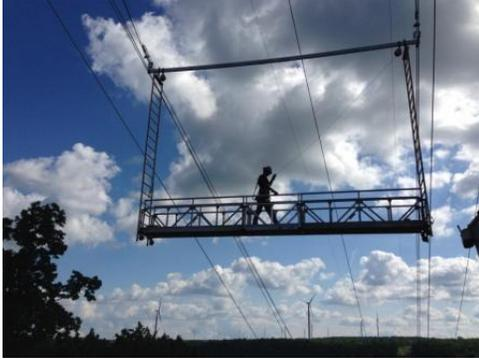
Seattle – Spider, a division of SafeWorks, LLC, provided a complete suspended access solution for the installation of spacers along conductor lines at Mehoopany Wind in Noxen, Pennsylvania.
