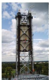
On site renovations took place nearly 130 feet above the roadway (200 feet above the river) with minimal existing walkways to access the work points. The ST-17 Air Spider was the perfect solution, allowing access throughout the project and requiring only a single rigging point.
