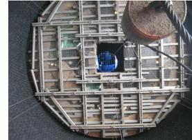
Spider’s professional engineers performed site visits in the process of designing a unique 31 ft round float platform equipped with nine SC-1500 traction hoists.
