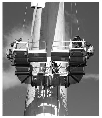
SA-1051 Flydecks can be added to ST-17 or ST-180 hoists or used to enclose Spider modular platforms such as the blade access platform pictured here.
