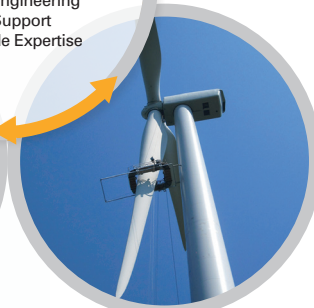
Energy (Wind, Nuclear, Oil & Gas)
